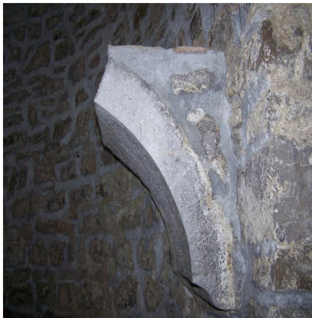
Picture 11-12. Elements architectural
